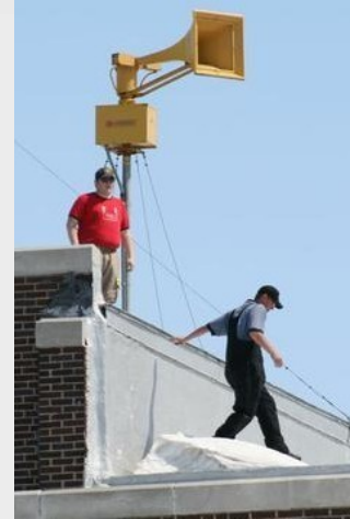
Fire department inspects a roof
